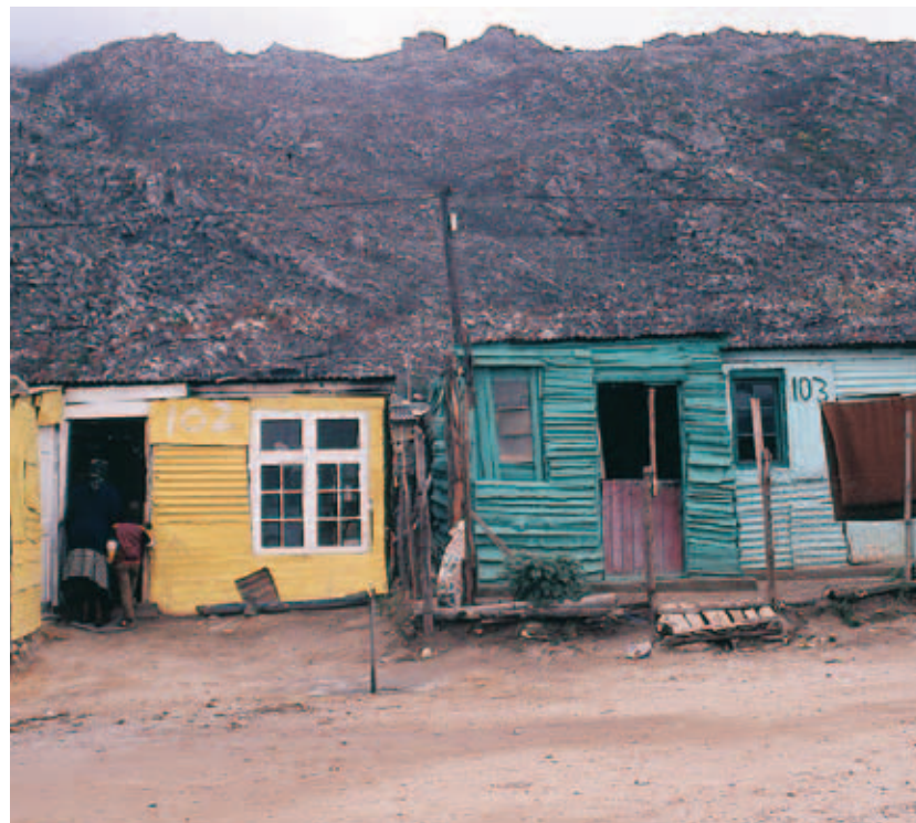
Yellow house on the corner.
